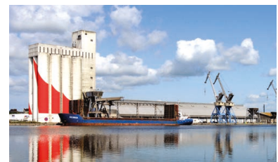
ESCAL'ATLANTIC, EOL (WINDZENTRUM), ÖKOMUSEUM, UNTERSEEBOOT ESPADON, SAINT-NAZAIRE
